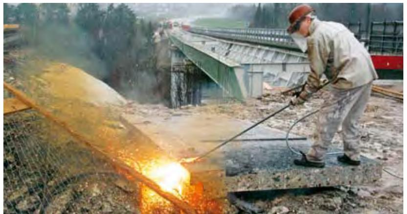
Concrete cutting with oxygen lances generates temperatures of up to 2,500 degrees centigrade.
