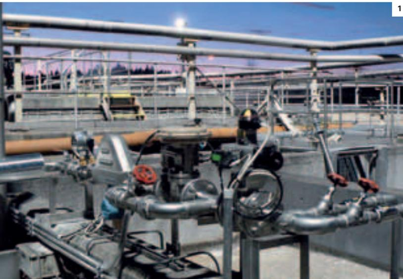
*1 State-of-the-art technology simultaneously provides for injection of oxygen and circulation of waste water in industrial effluent treatment plants.*
