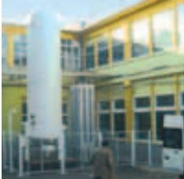
*Kuhnke in Romania uses liquid nitrogen for inerting during the soldering of electronic components.*
