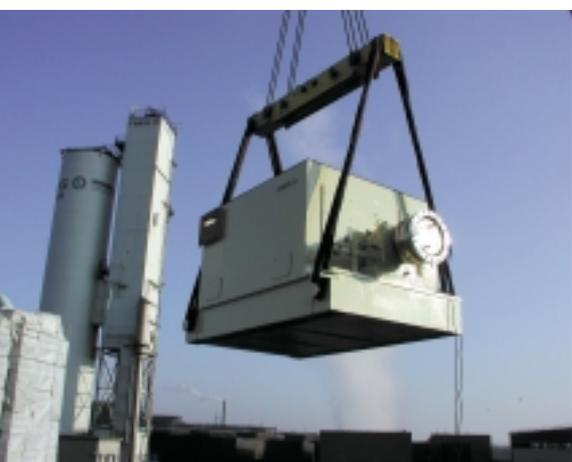
Delivery of the drive motor for the air separation plant in Dillingen
